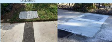
Chambers house important network equipment. The above shows the Chamber in a temporary state with black asphalt surround and in a permanent state once the network is complete.
