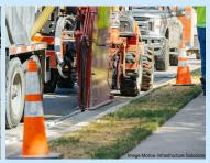
Cutting a trench for the fiber conduit.
